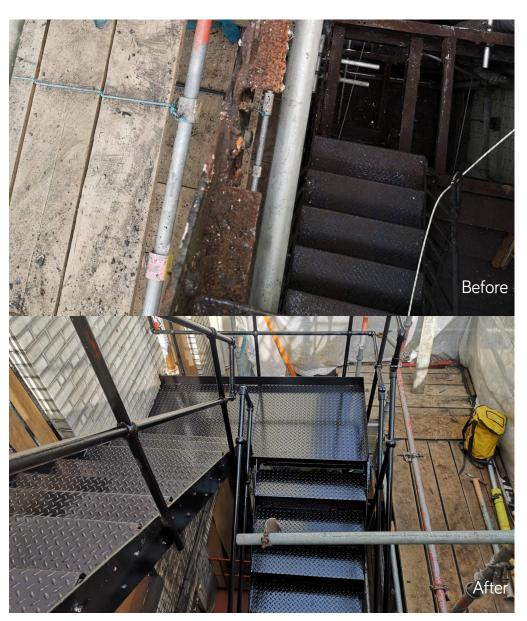
Premier Technical Services Group Ltd (PTSG) has completed a specialist rope access project at an office building in Strathclyde, replacing a large steel fire escape.
