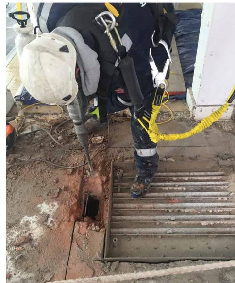
‘This was the first time some of the tower’s steel had been renewed or replaced, and crucial sections had corroded over its 125-year life span’
