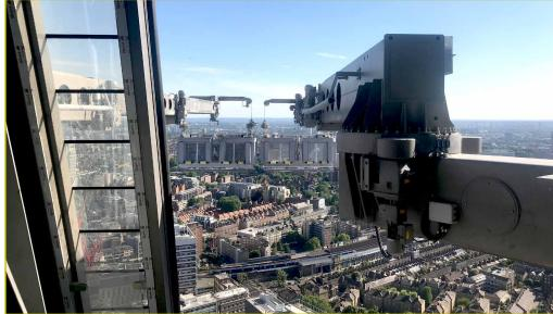
Each skyscraper requires its own unique access system and The Vase is no exception. Integral Cradles installed three building maintenance units, which were fitted to integrate with the building's moving doors – also designed and supplied by Integral Cradles, to carry the intricate cladding panels and mask the garage area. This allows the BMUs to be concealed without any visual sign of the systems.
