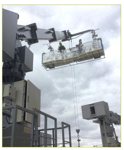
8 Canada Square is the global headquarters of HSBC Group, a 45-floored skyscraper standing 200 metres high. When two of the building's maintenance units (BMUs) became defective, PTSG's London-based Access and Safety division, Integral Cradles Ltd, was commissioned by HSBC to replace the existing units with warrantied replacements.
